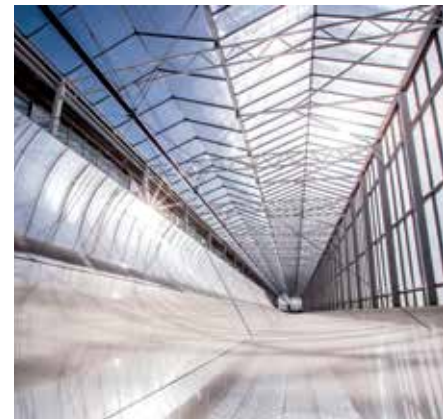
The world-leading Miraah solar project
