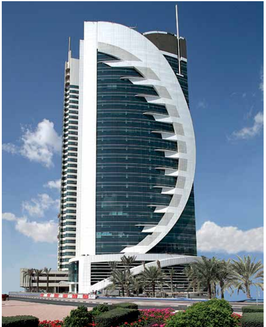
Doha Bank tower
